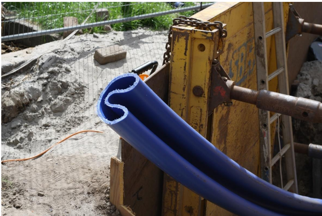
Figure 2 Application of Compact Pipe in Zwaagwesteinde, Friesland.
