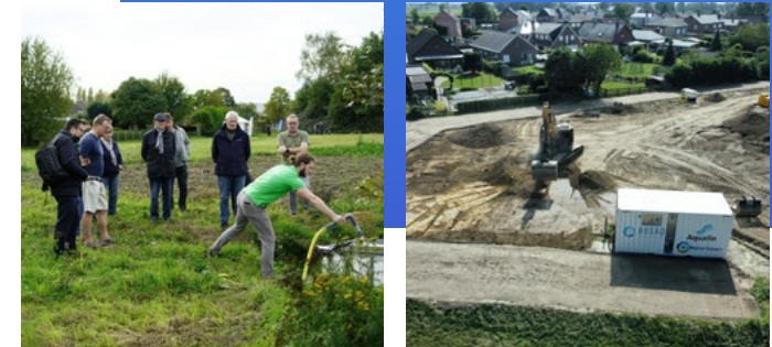
Left: Local event: Pumpkins for citizens Right: Construction of the buffer basin in Mechelen
